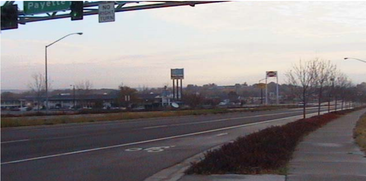
Figure 5. Picture Showing Existing Conditions – Curb/Gutter, Raised Median, Bike Path
