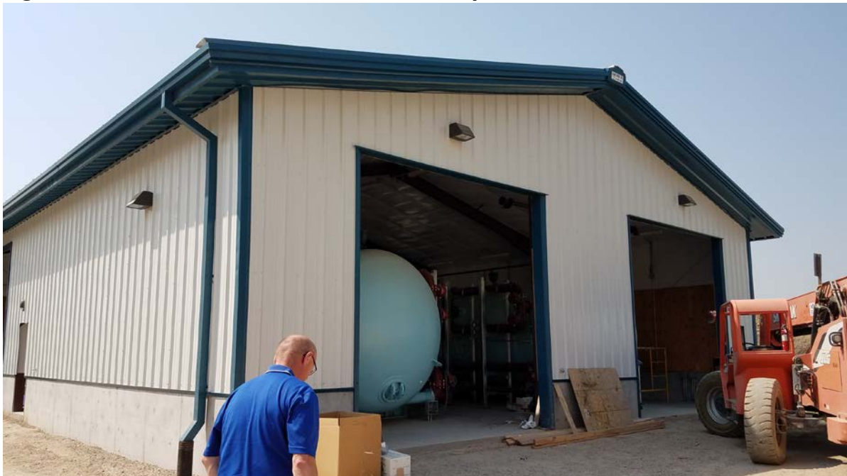
Figure G-2 View of the Water Treatment Facility
