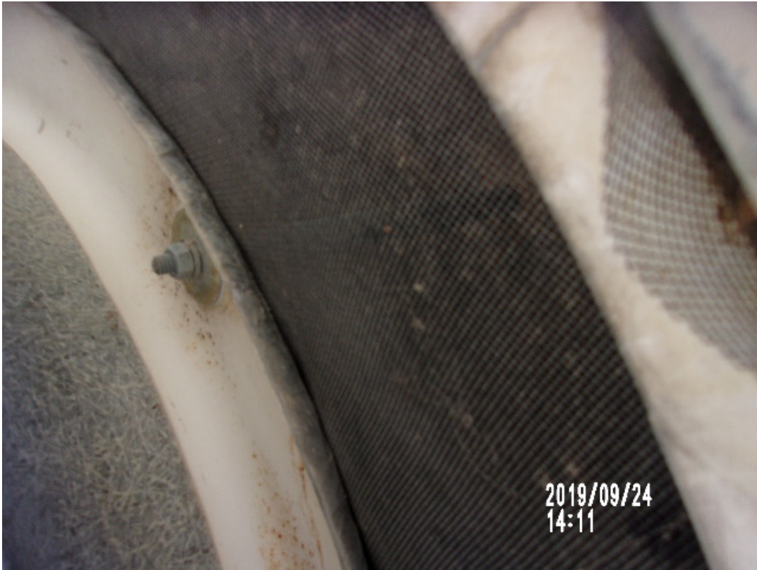
Roof Vent Screen
