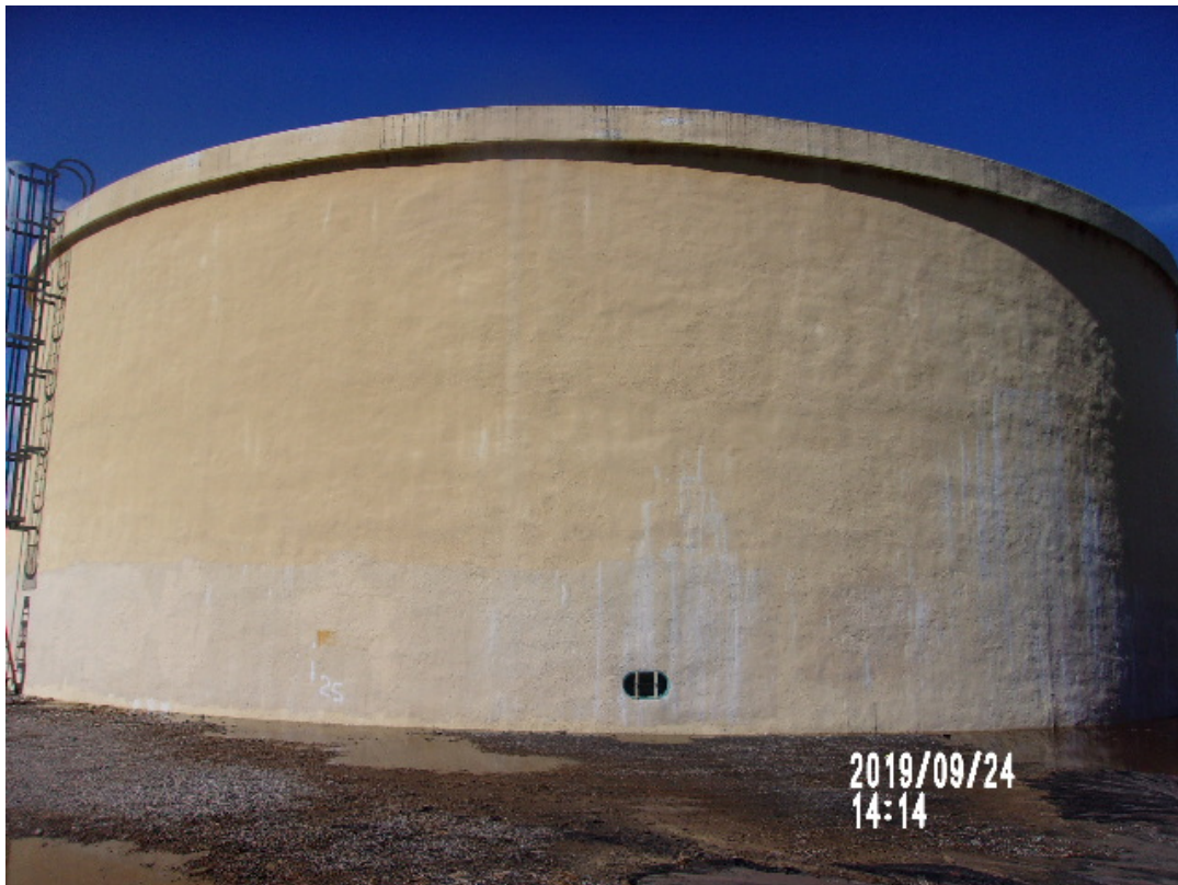
Exterior Reservoir and Man Entry
