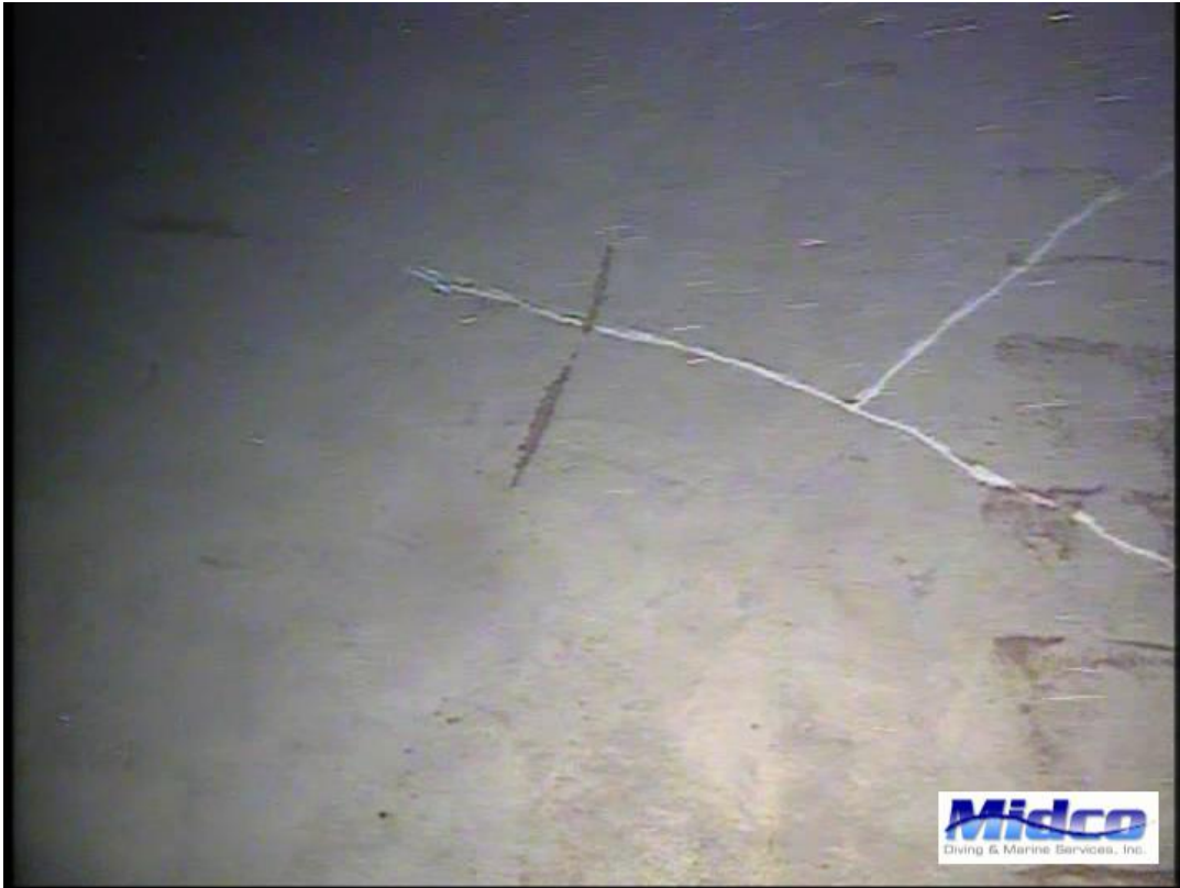
Typical Floor – Settling Cracks with Previous Repairs Noted
