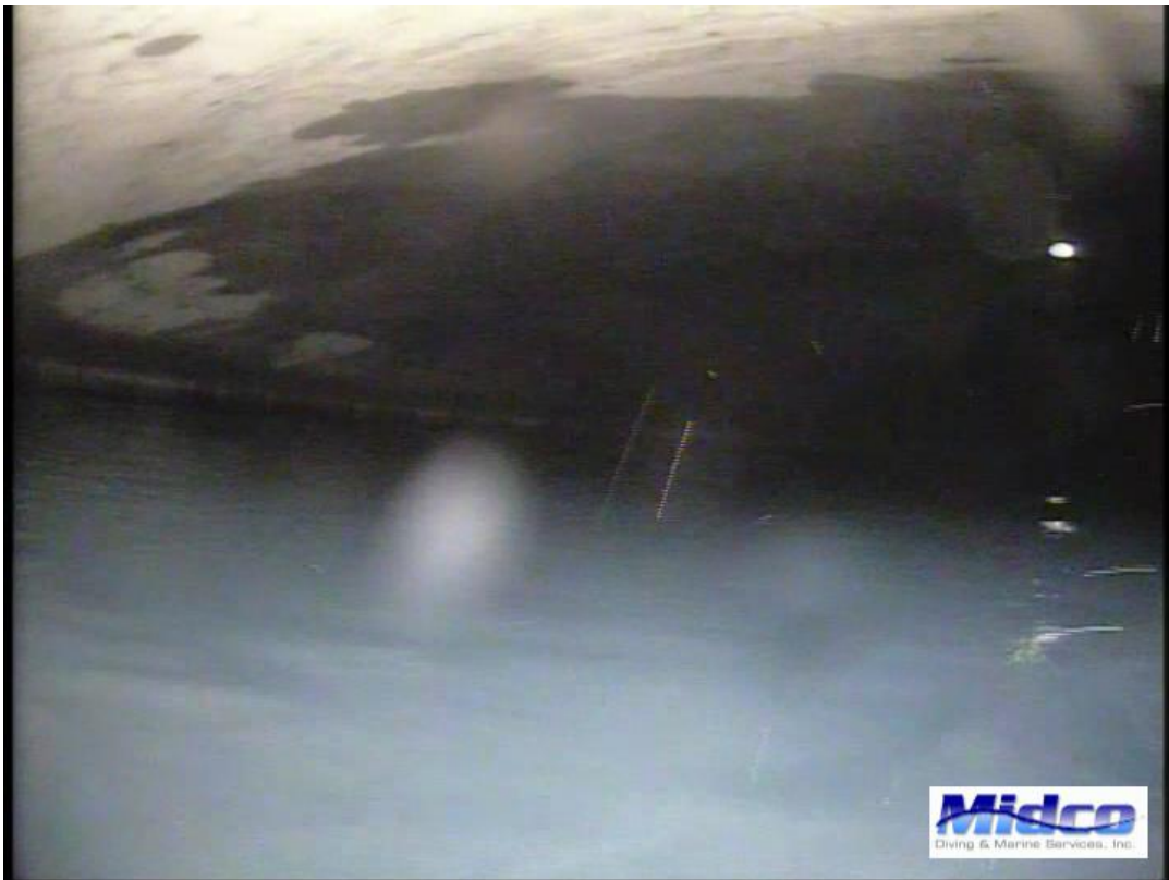
Typical Roof and Vent
