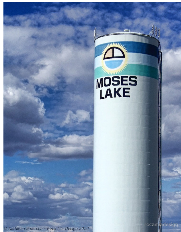
Standpipe Style Welded Steel Reservoir Moses Lake, Washington (courtesy of Rocamia Design)
