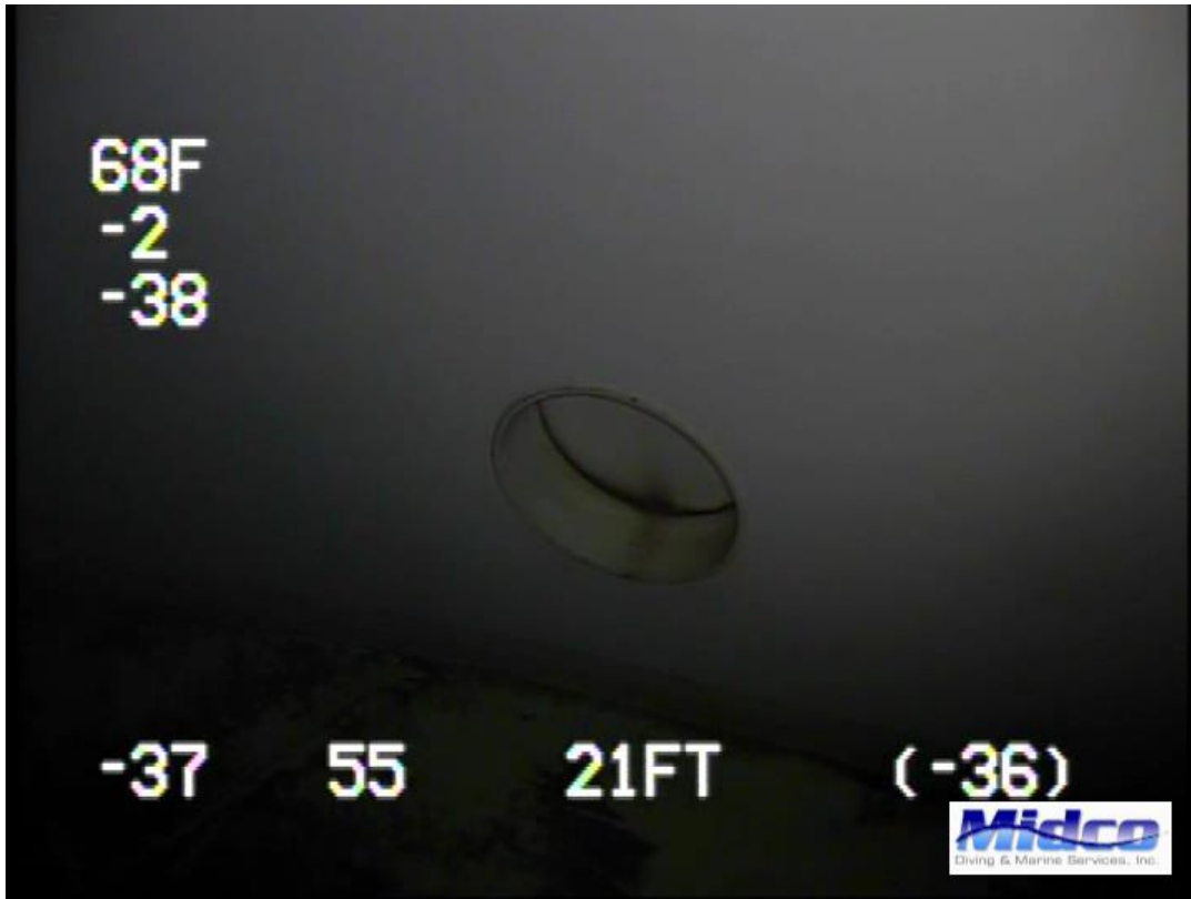
Second Man Entry – Coating Failure with Corrosion & Staining Noted
