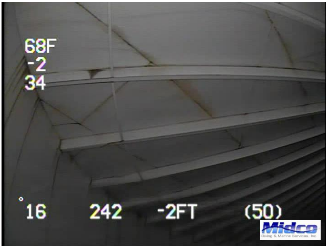
Wall to Roof Seam
