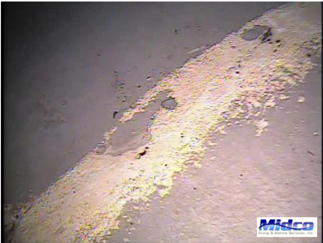
Typical Floor – Settling Cracks with Previous Repairs Noted
