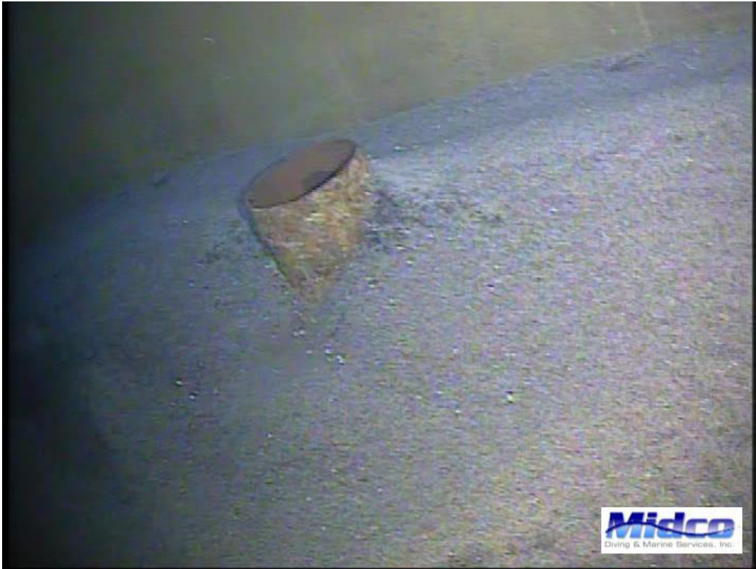
Up to 21" of Sediment Noted Near Inlet Plumbing – Possible Filter Rupture
