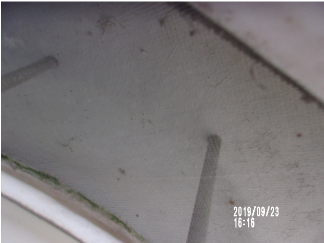
Roof Vent Screen
