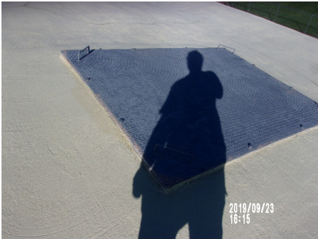
Secondary Access Hatch
