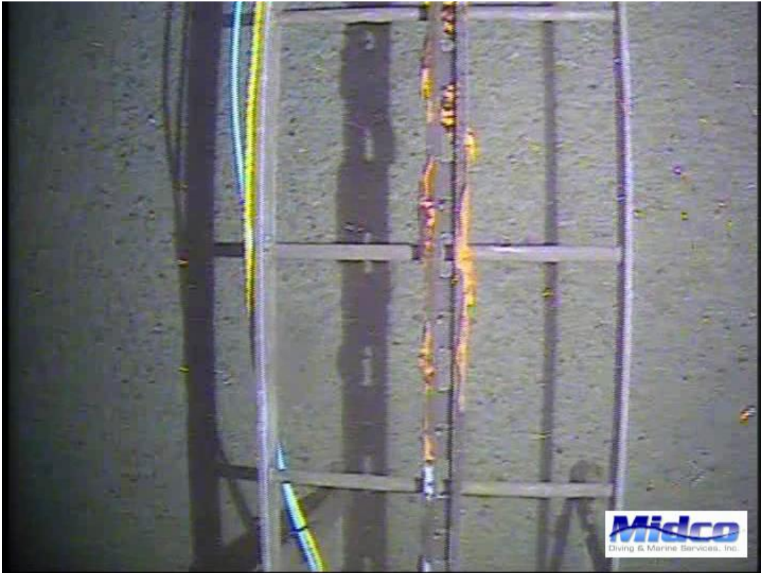
Interior Ladder and Safety Rail
