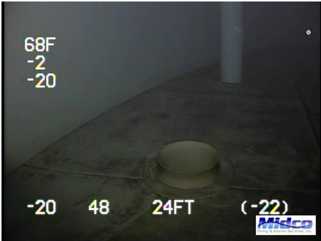
Second Man Entry – Coating Failure with Corrosion & Staining Noted
