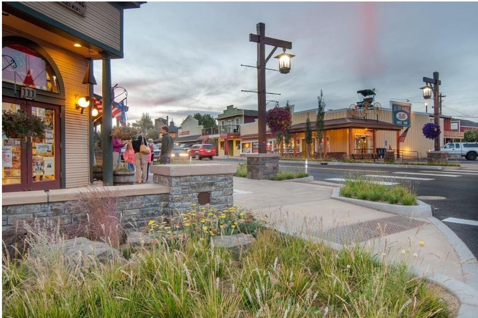
Native plants in stormwater infiltration planter
