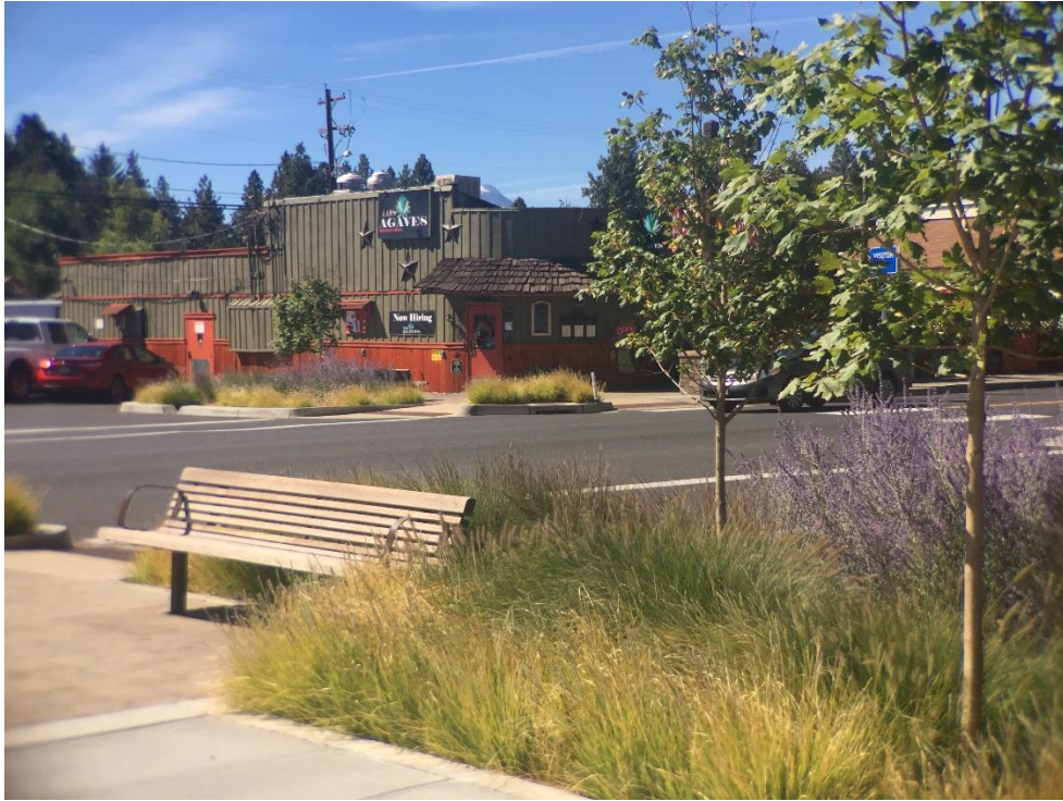
Bench at stormwater infiltration planter
