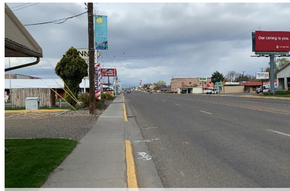
Curb-tight sidewalk on SW 4 th Avenue
