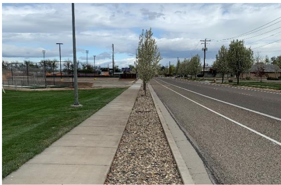
Buffered sidewalk on SW 4 th Street
